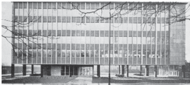
fig.200: Irish Life building, Mespil Road, 1960's
